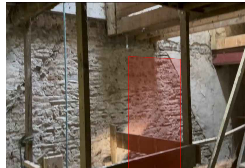
03 Image of Existing wall of the location of Intervention 06 Scale: 1:20
