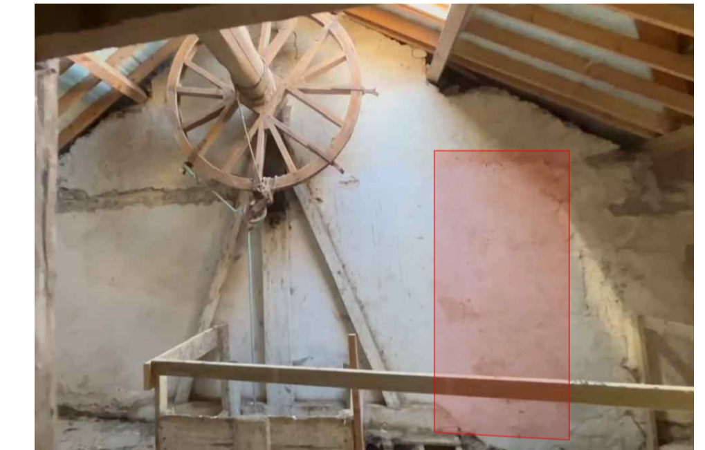
07 Image of Existing wall of the location of Intervention 07 Scale: 1:20
